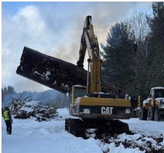
The culvert is OUT! —Photo taken on Monday, December 2, 2024 at 2:30 pm
