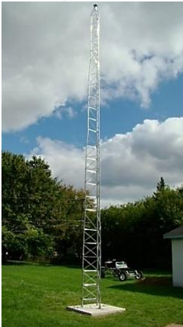
Pictured here is a typical repeater installation. Raven Hill is planning an 8' wooden guard around the bottom of our tower, just to keep kids safe--no climbing allowed!
