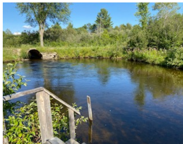
View of the Fuller Road culvert from Viewing Platform
