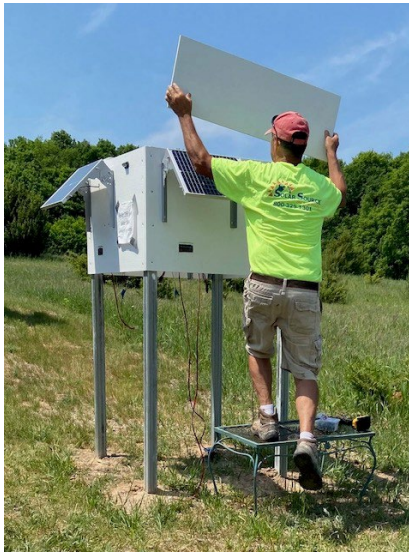
Paul Cusack of West Michigan Solar continues to problem-solve and make progress on the Solar SMART kiosks, which will demonstrate the effect of direction and slope on the energy input from the sun.
