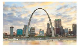
The arch's two legs were built separately, and if their measurements were off by as little as 1/64th of an inch, they would not have been able to join at the top.
