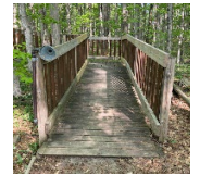
The Treehouse ramp looks as good as new, after several trees fell on it during a winter windstorm.
