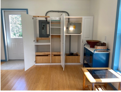
Open cupboard doors show off the storage batteries below with the inverter and circuit panel above, all used to capture the solar energy used to lay the bamboo floor seen in the foreground.
