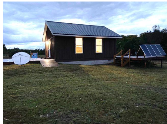
Using the existing solar panels at the Energy House, evening visitors can fix food and listen to music, in addition to enjoying the new Solar SMART lighting— all compliments of our funders and the sun!
