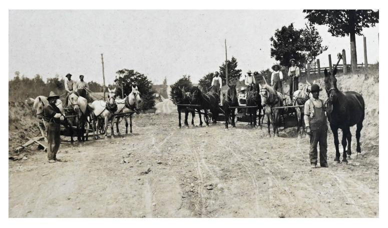
Road construction taking place in the Boyne Area. A five-double team horse-drawn Wheeled Slip/Pan Road Scraper is being used.
