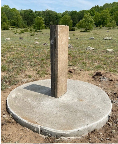
Now, the Altar Stone at Raven Hill stands vertically welcoming positive energy to the Center's many visitors.
