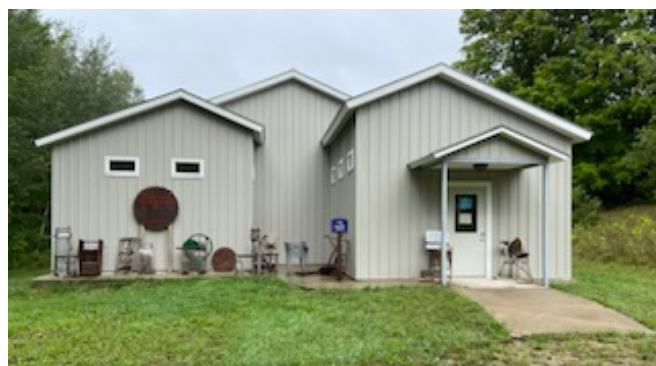
Built in the shape of a capital “H” for History, the ET allows visitors to view changes in technology from the Stone Age to the present.
